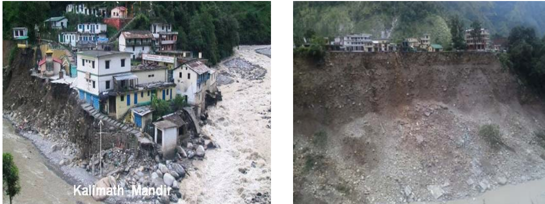
Fig. 1: Damaged Kalimath Temple in Distt. Rudraprayag and Buildings in Distt. Pithoragarh
