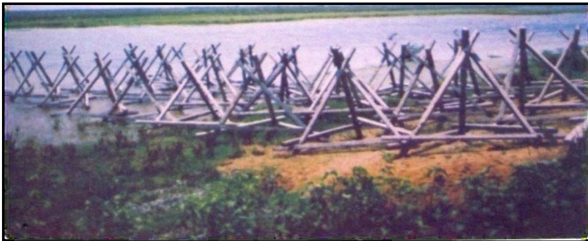
Figure 2: RCC Porcupine Spur
