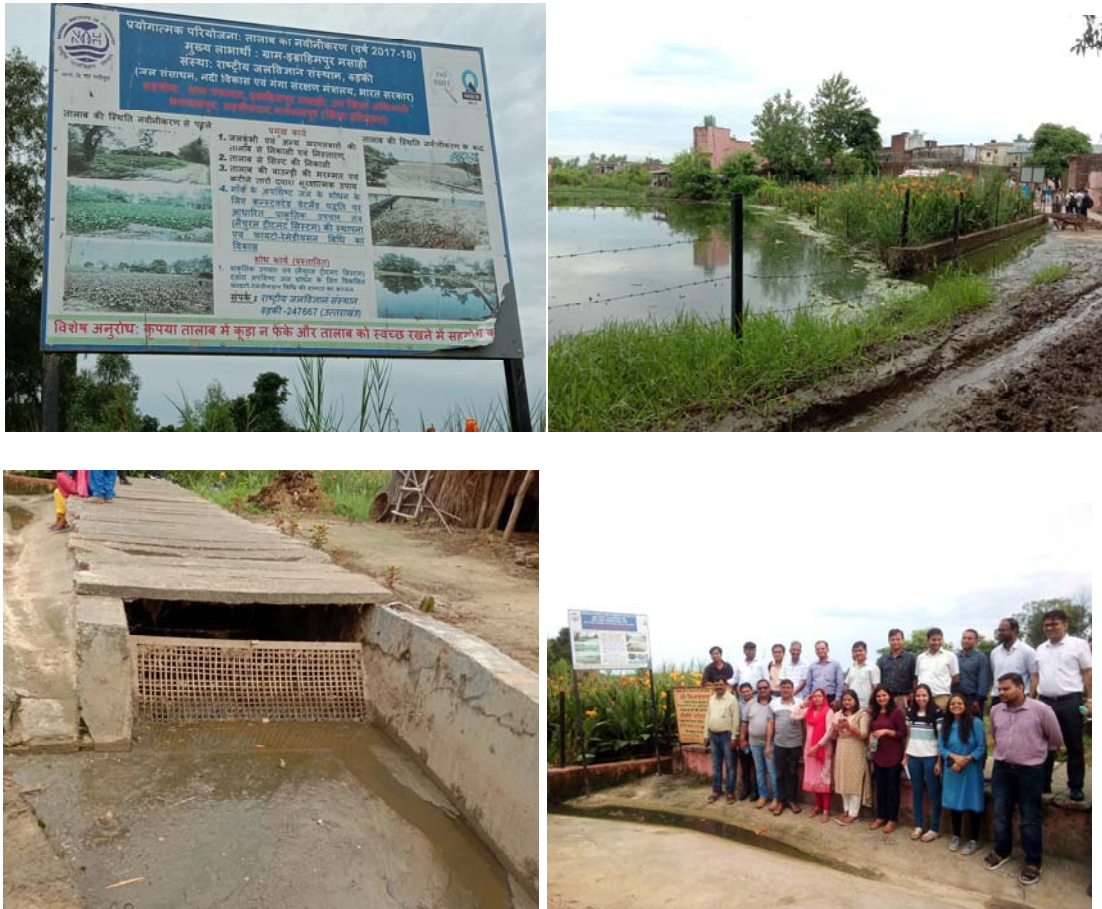
Field Visit to the Constructed Wetland at Ibrahimpur Village in Haridwar, Uttarakhand
